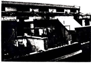
Raising the roof and adding one story, plus interior improvements, produces increased accommodation at better standards with more sunny and usable space, at Lane 303, Peng-Lai Road, Shanghai, built in 1923.
