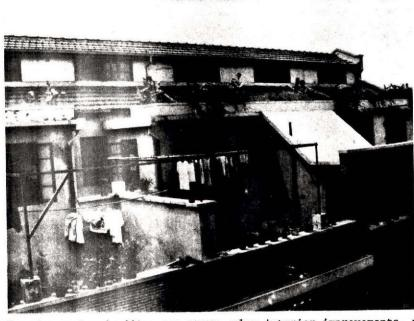
Raising the roof and adding one story, plus interior improvements, produces increased accommodation at better standards with more sunny and usable space, at Lane 303, Peng-Lai Road, Shanghai, built in 1923.
