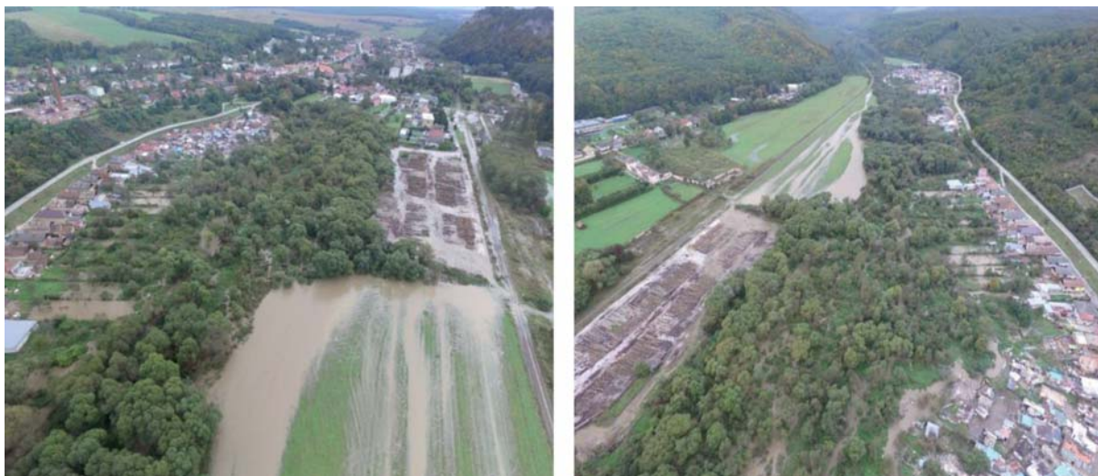
FIGURE 2. Drone photographs of flooded area of Roma settlement in Jasov, 2020
