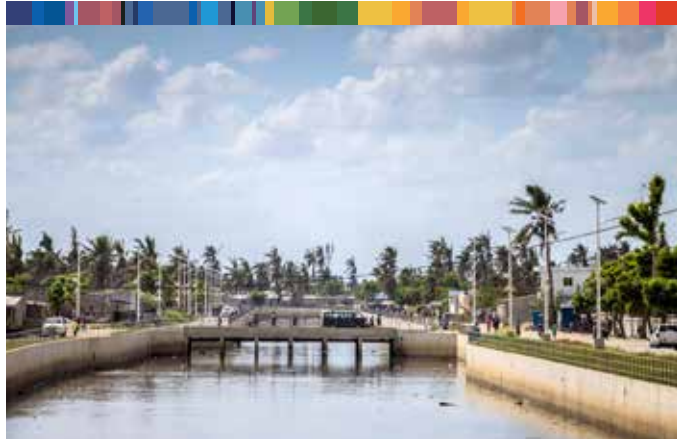
A stormwater drainage system that helped build resilience in Beira, Mozambique. Resilience-building interventions in the city, including implementing nature-based solutions, helped the city manage the impacts of Cyclone Idai in 2019. –PHOTO BY SARAH FARHAT / WORLD BANK
