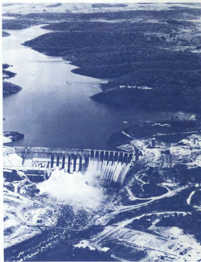
The Guri Dam in Venezuela also received World Bank assistance.
