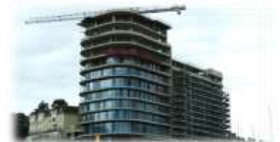
Buildings (e.g. University campus)
