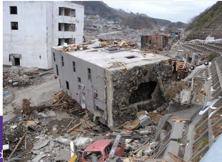
Destruction on building at Onagawa
