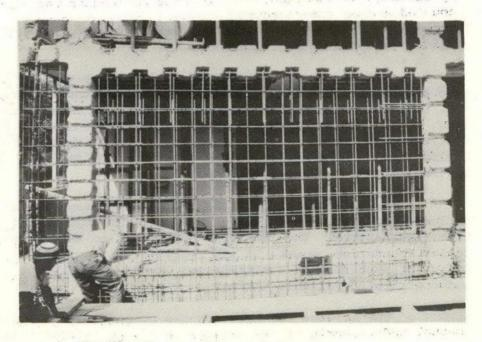
Repairs to provide a rigid wall structure
