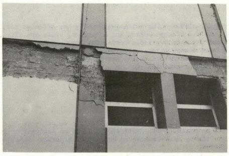
Example of earthquake damage to CIP headquarters The central column in this picture is the righthand column in the picture below
