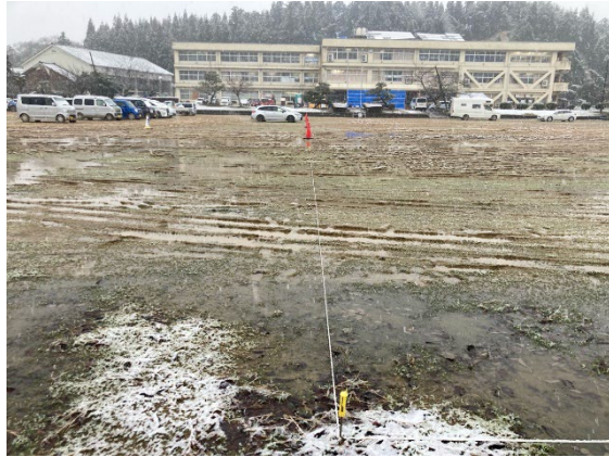
Before construction begins
