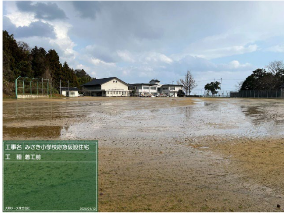
Before construction begins
