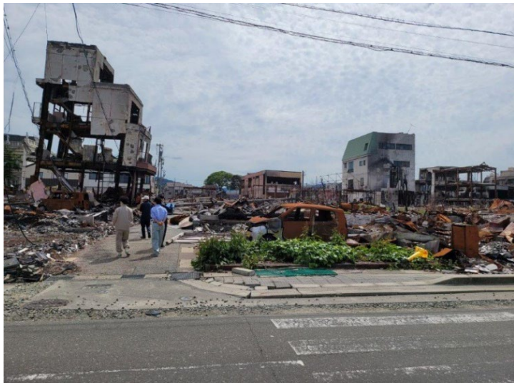
Fire damage Wajima Morning Market (Wajima City)
