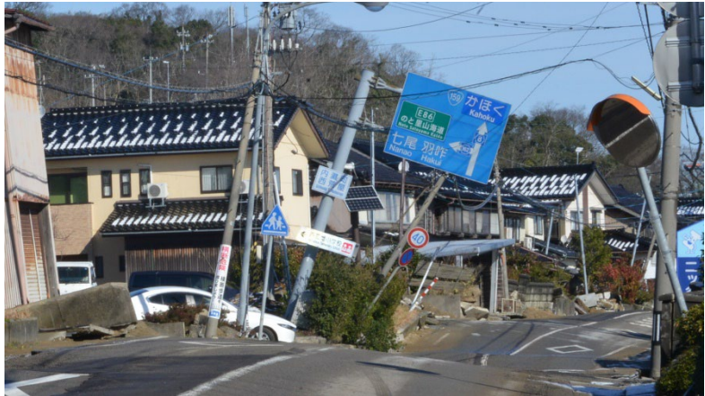
Liquefaction, lateral flow (Uchinada Town, etc.)
