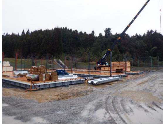
H steel foundation
