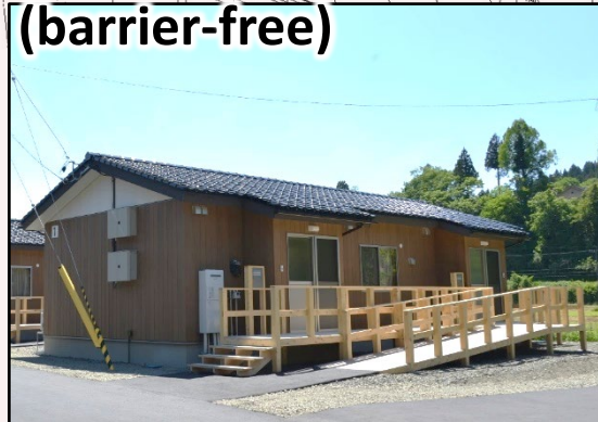
Installing ramps and outdoor corridors
