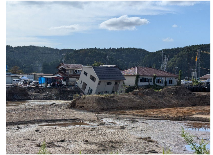
River flooding and levee destruction (Wakayamacho, Suzu City)
