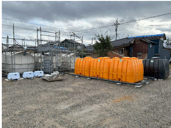
Water tank/septic tank
