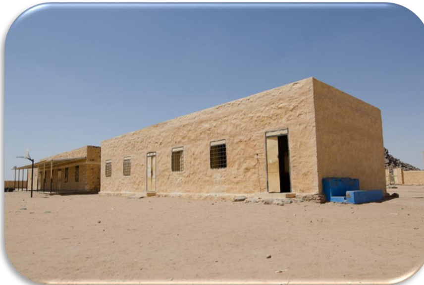
Two new class rooms built by the CDF at Manan Telkoug, Kasala to expand the school - Sudan
