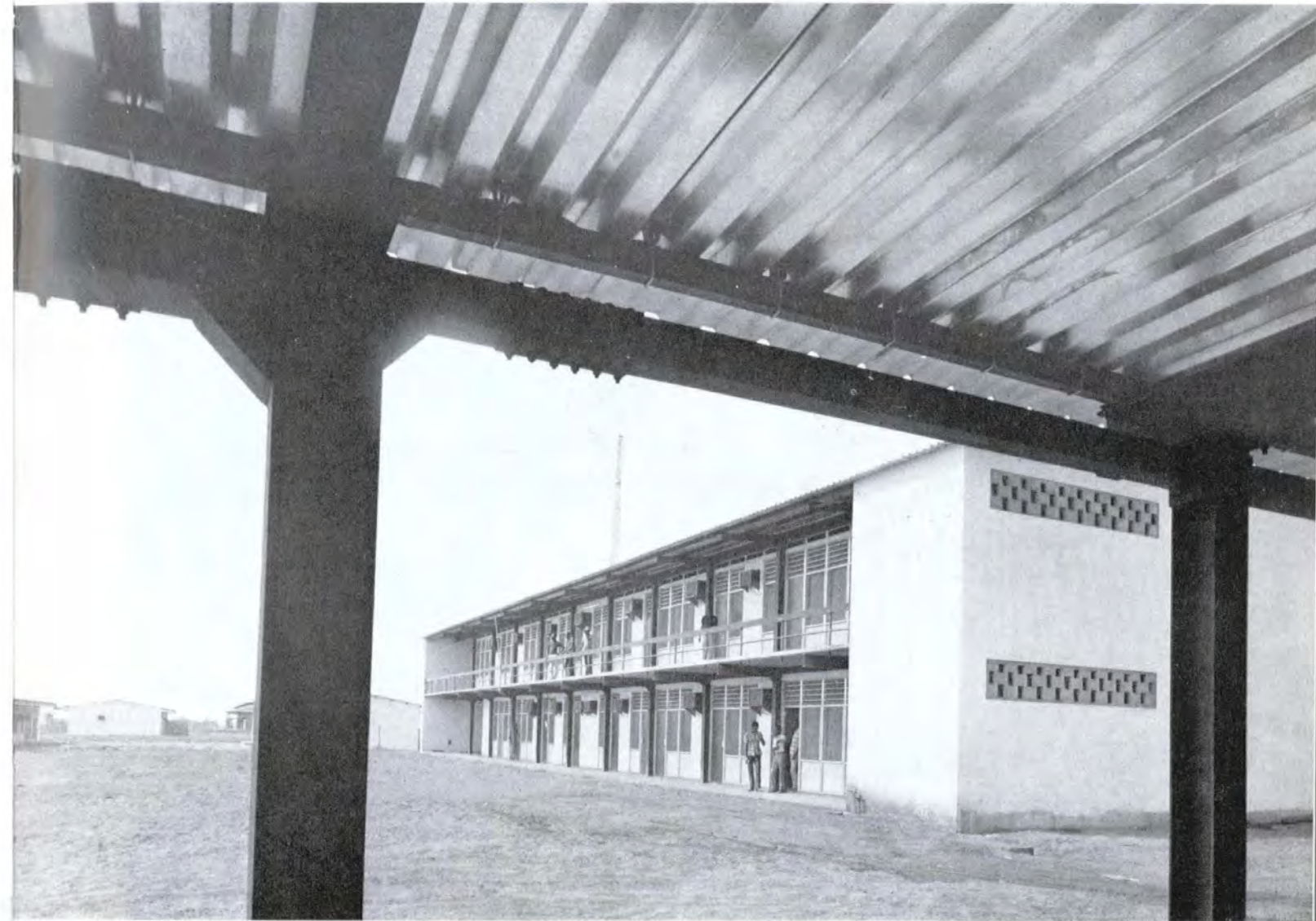
Administration Building at Kamsar.
