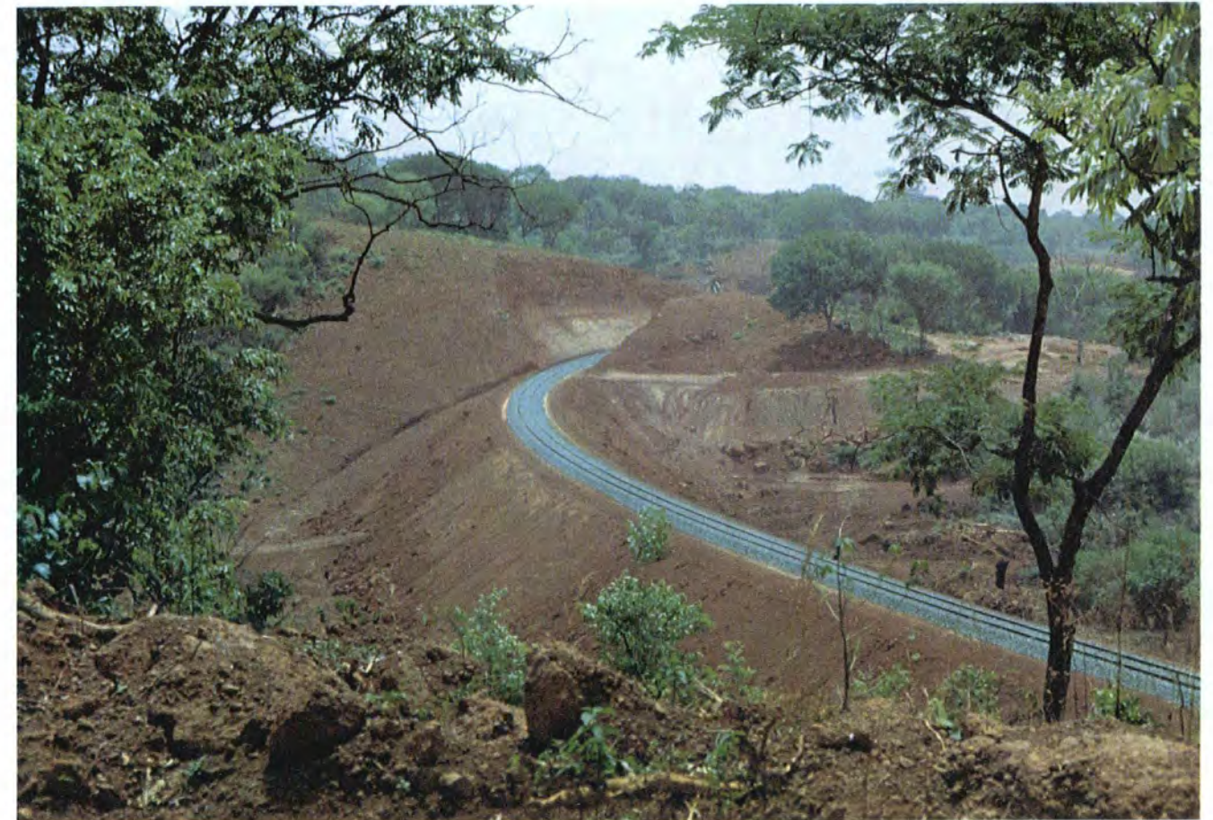
Earthmoving along Sangaredi - Kamsar railroad line.
