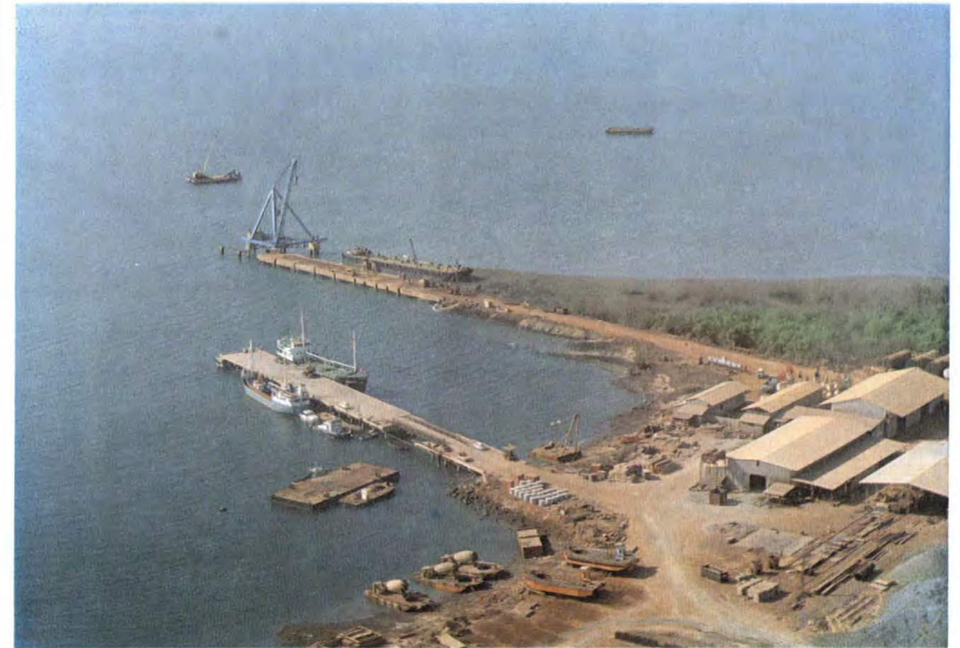
The Port of Kamsar (under construction).
