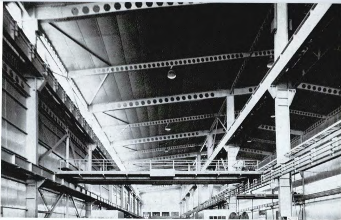
Repair and maintenance workshop (indoor view).
