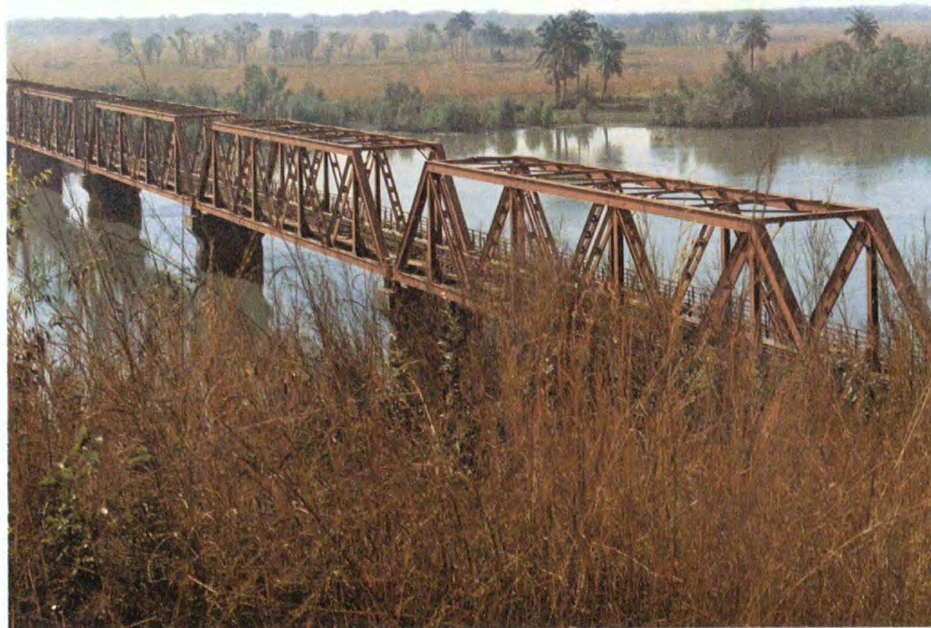
Steel bridge on the Rio Nunez.
