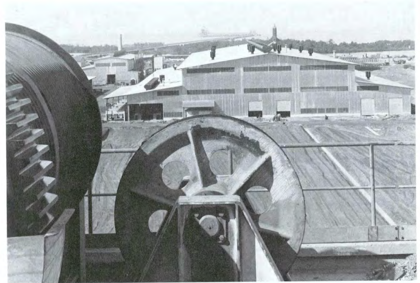
Repair and maintenance workshop.
