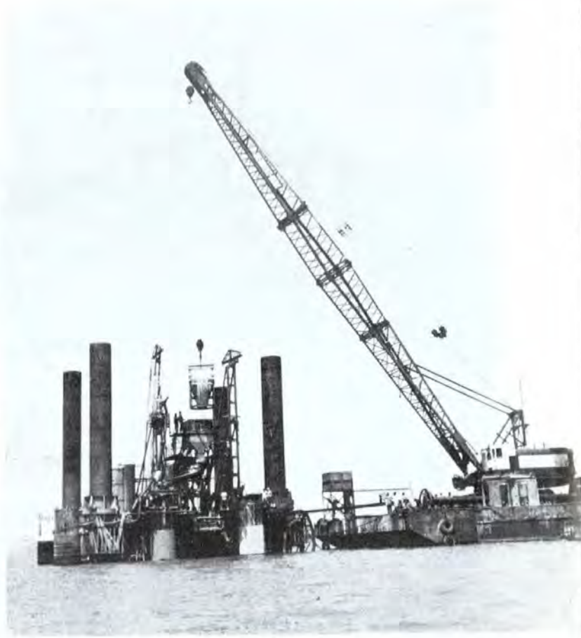
Pile boring pontoon.
