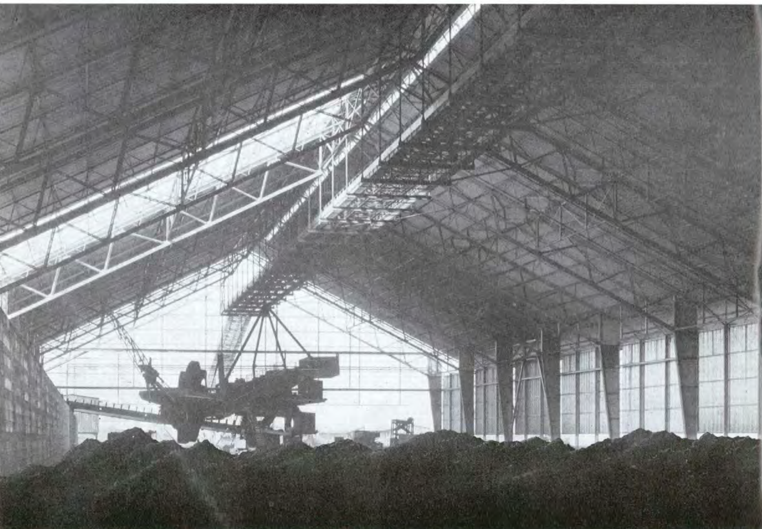
Bucket wheel reclaiming dried bauxite in the storage hall.
