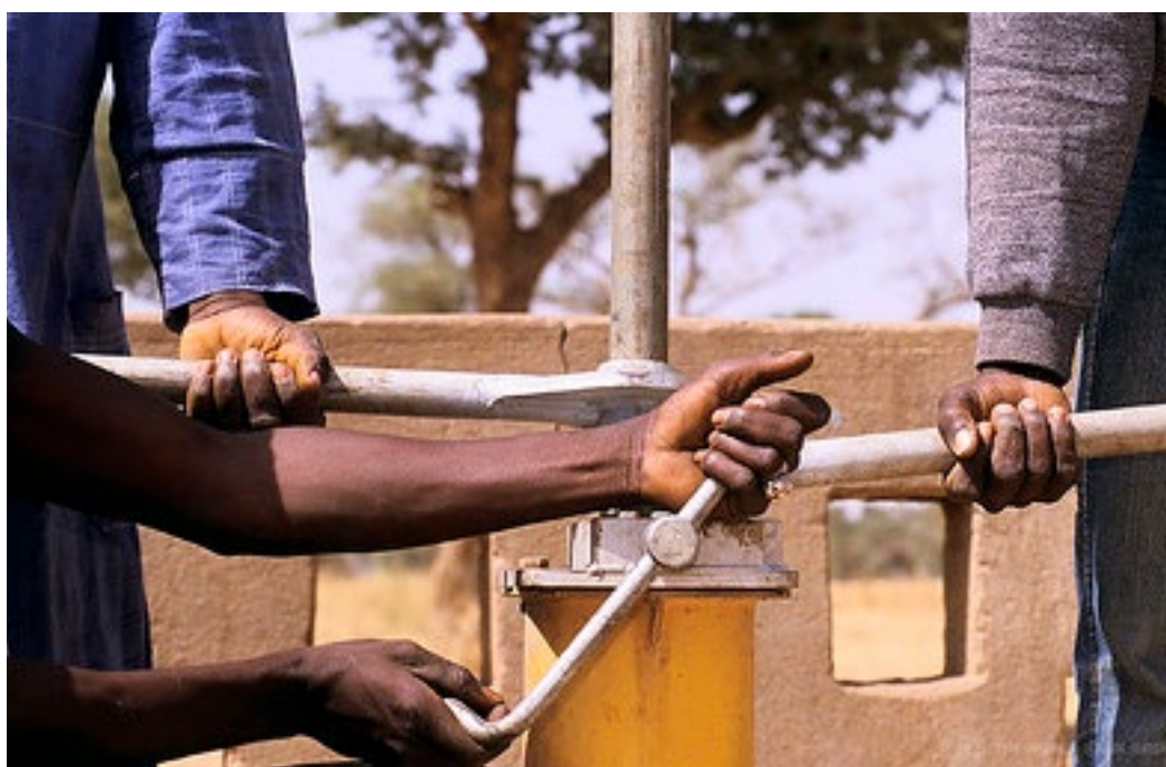
Building a water pump in Mali.
