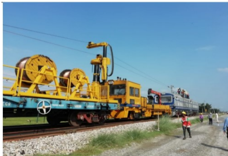
NOTE. Process of Electrification
