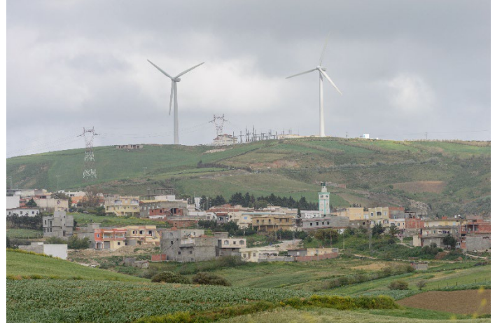
Figure 1 Wind turbine in Northern Tunisia Photo Credit Shutterstock by Mashhour
