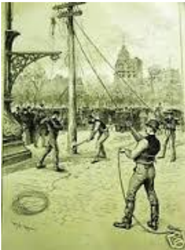
Figure 53: Removal of telegraph and telephone poles and lines in New York City in 1889
