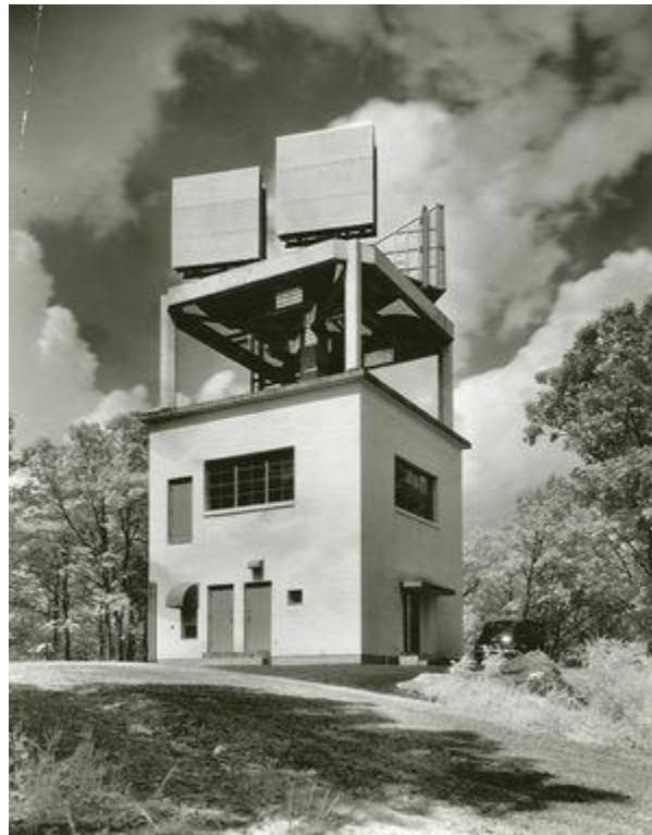
Figure 10: Microwave tower used in first commercial long distance telephone relay system
