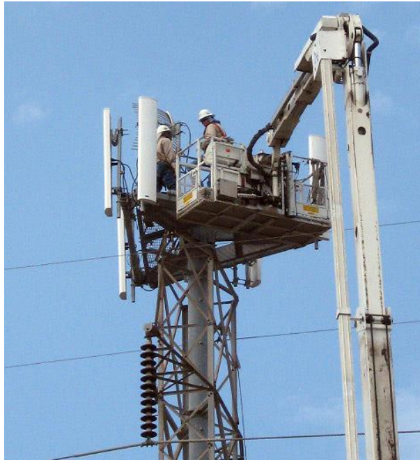
Figure 13: Installation of cellular antenna on electric transmission tower
