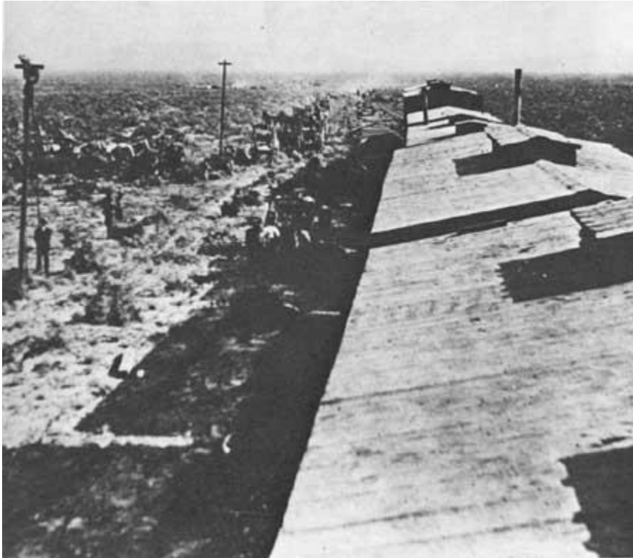
Figure 50: Installing the telegraph lines on poles along the railway
