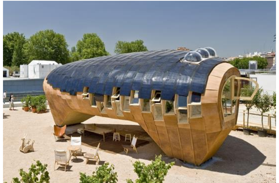
The Solar House
