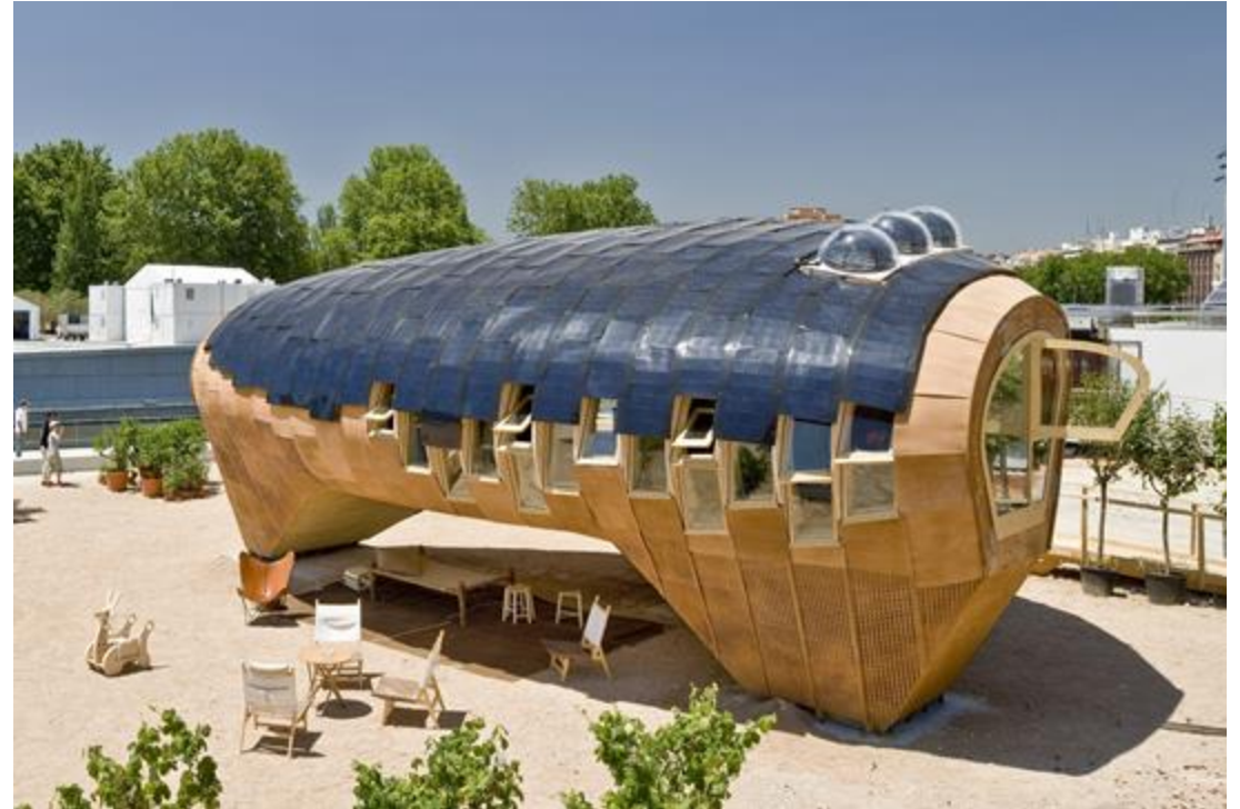
The Solar House
