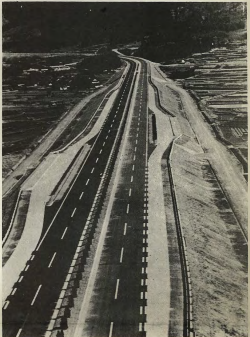
The Nagoya-Kobe Expressway near Kyoto, Japan, where the Yamashina project's first strip of test pavement in asphalt measures 4,300m. in length. The 5m. high embankment is widened to accommodate bus stop lanes
