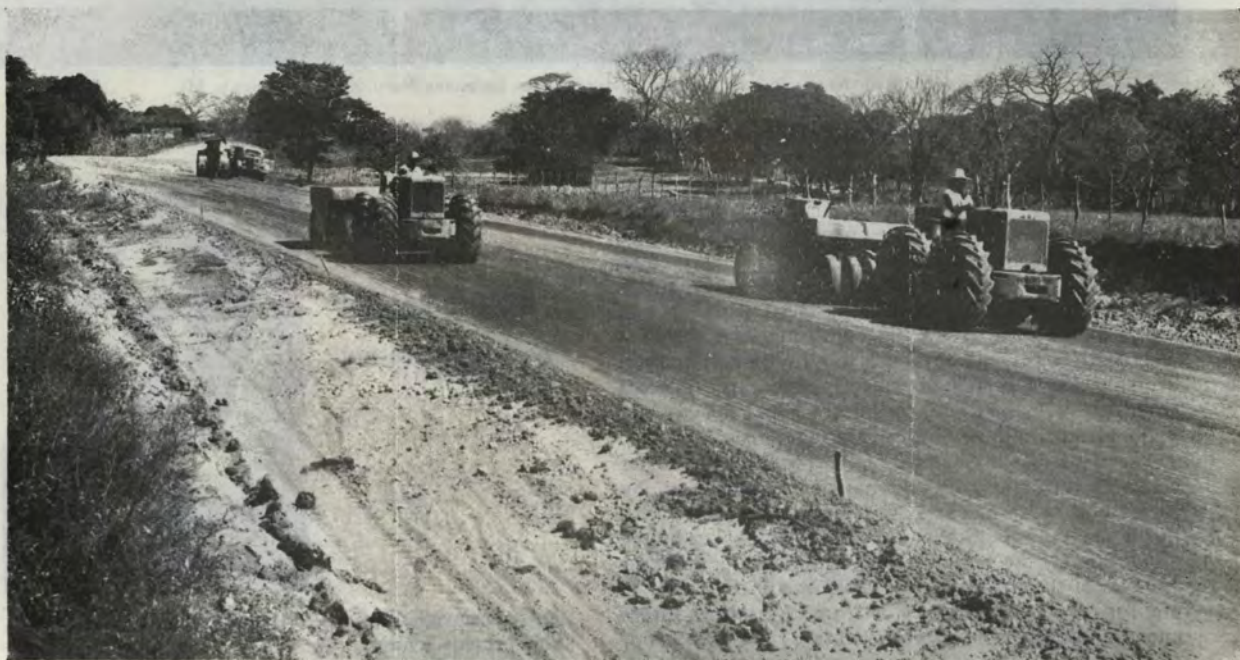
Compacting the base of the Granada-Masaya highway, Nicaragua, another I.B.R.D. project
