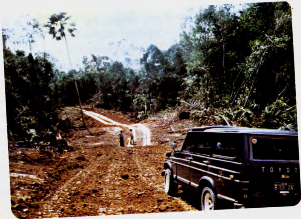
NEW VILLAGE ROAD UNDER CONSTRUCTION
