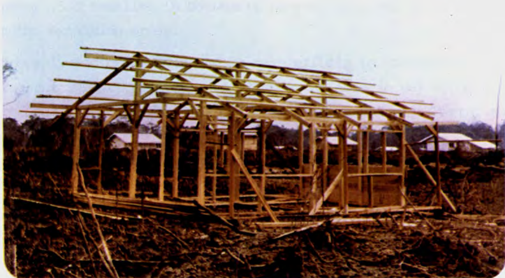
BASIC WOODEN STRUCTURE OF A TYPICAL TRANSMIGRANT HOUSE
