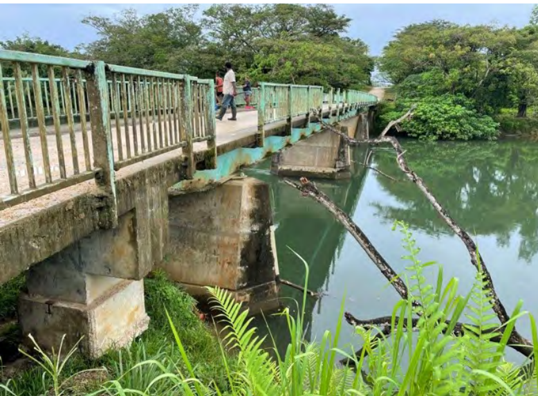
A bridge on South Santo Road, Vanuatu. © Dung Anh Hoang/World Bank
