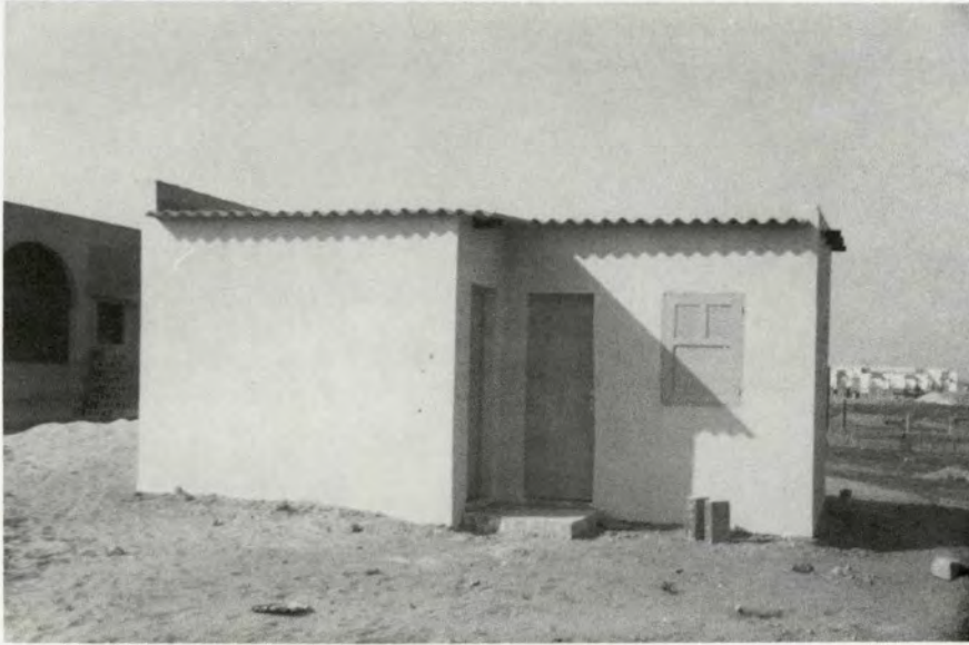
A typical two room unit ready for occupancy.
