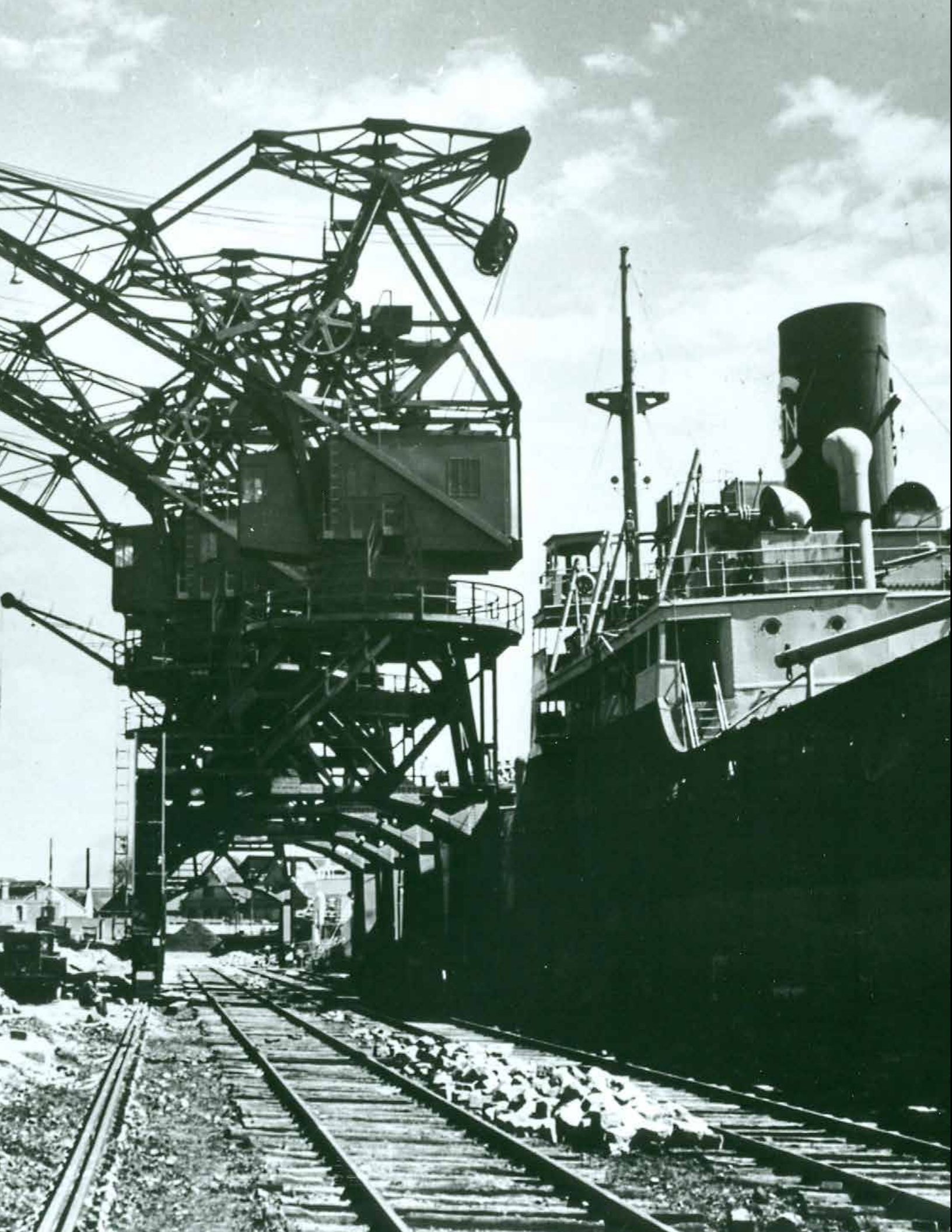
Opposite page: Equipment near a railroad tracks, France.
