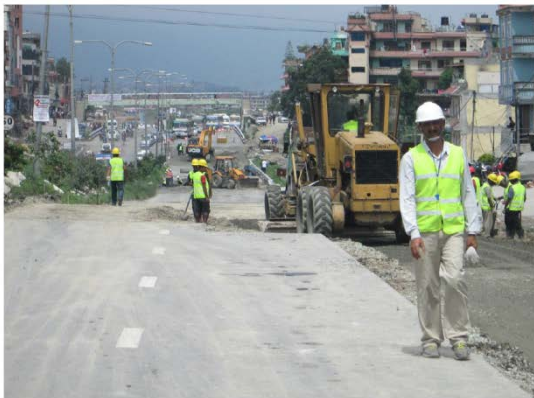
Eastbound Lane Base Coarse Laying July 20, 2015
