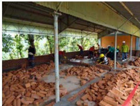
Repairs progress at a rapid pace.
