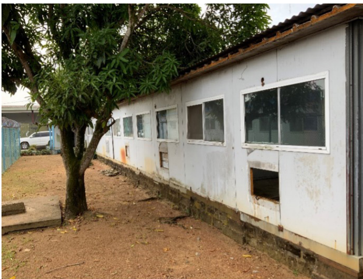
Non-rehabilitated Structure at the COVID Treatment Center
