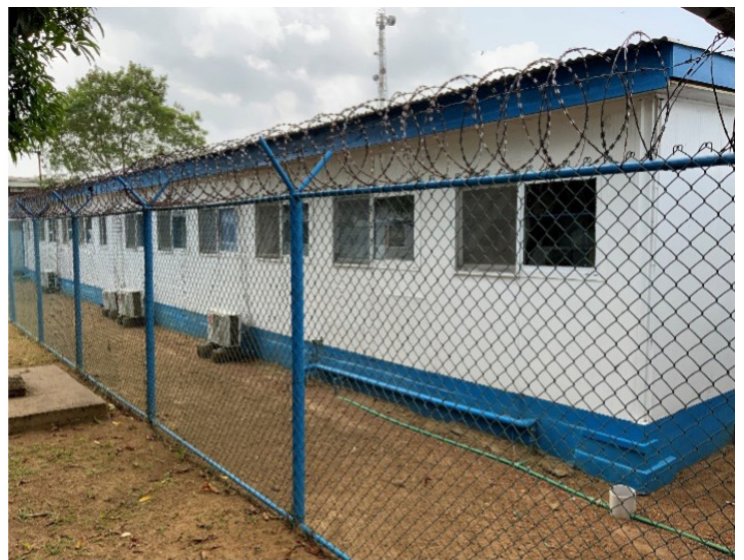
Rehabilitated Structure at the COVID Treatment Center
