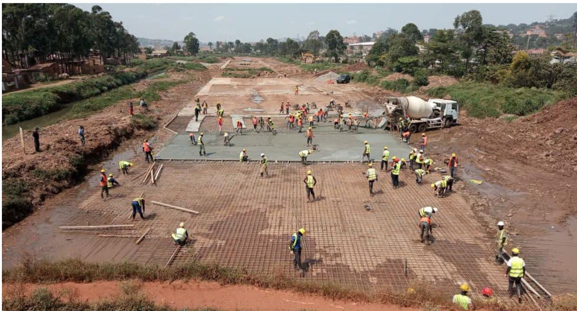
*Picture 6: Silting of the Lubigi channel is being addressed through concrete lining of the channel in the Bwaise-Kawaala section where the works are ongoing (this is not the Kawaala-Hoima Section which pertains to the Request).*
