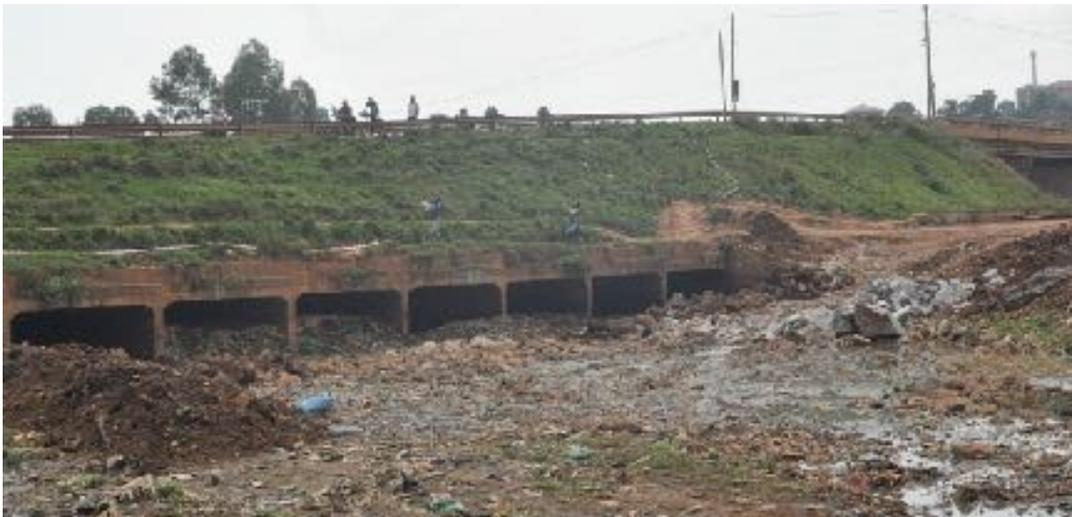
*Picture 5: Silting of the box culverts at Kawaala Bridge (2021).*
