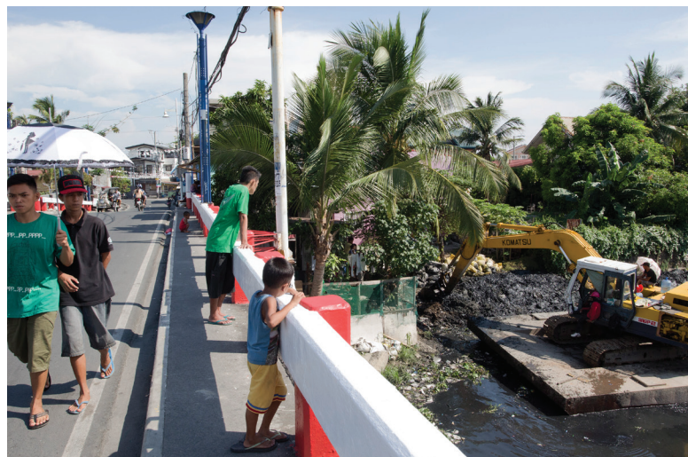
Pedestrians watch as city workers dredge the riverbed of the Taguig River; Philippines on July 11, 2014. Photo © Dominic Chavez/World Bank.
