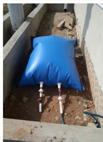
Gas produced from the biogas plant and ready for use. © World Bank.
