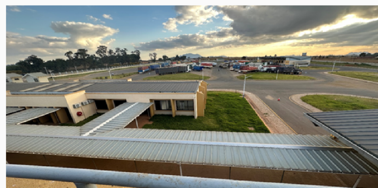
Photo: The Dedza One Stop Border Post Project constructed under the Southern Africa Trade and Transport Connectivity Project.
