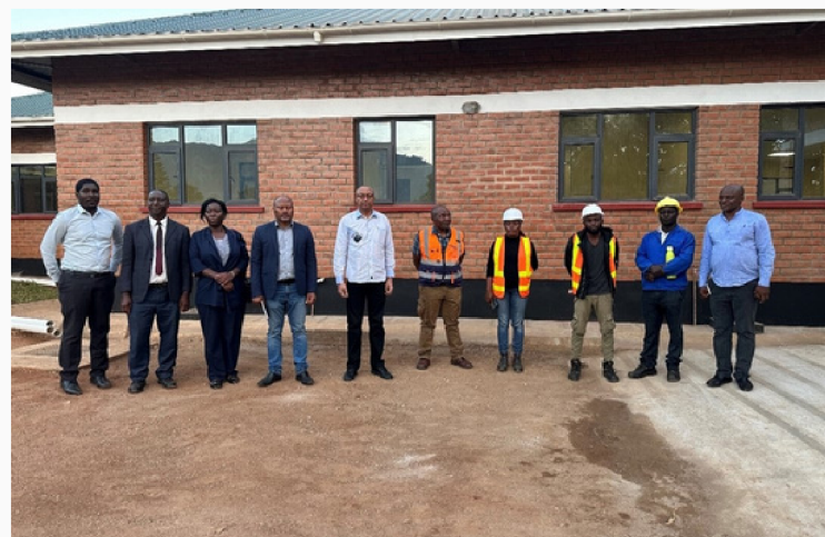
Photo: The Executive Director, Dr. Floribert Ngaruko with team of Engineers witnessing the 90% completion of the Dedza District Hospital with the support from the WBG.
