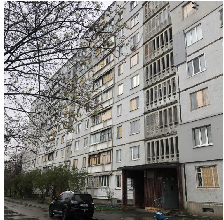
Druzhby narodiv, 227 Light damages Number of units – 126
